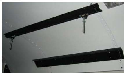
Figure 4-17 - Side Mount Evaporator Brackets
